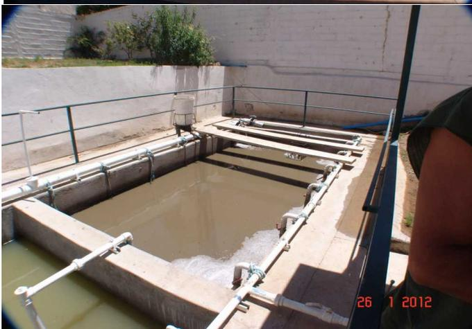
Sewer treated with EcoFlush and EcoGrease in oxidation tank.
