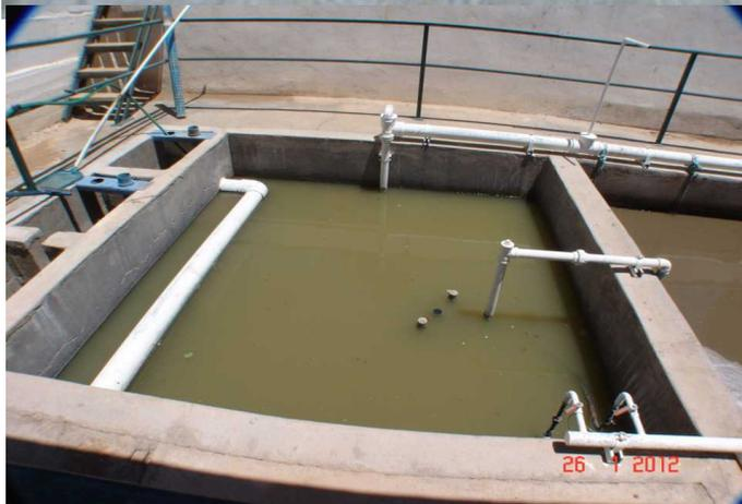
Sewage treated with EcoFlush and EcoGrease in sedimentation tank.
